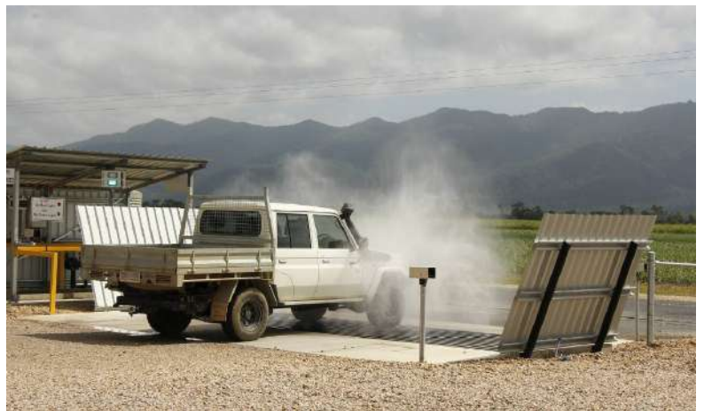
A vehicle and equipment wash down bay provides protection against soil-borne pathogens and hitchhiker pests. Credit: Queensland Department of Agriculture and Fisheries (QLD DAF).
