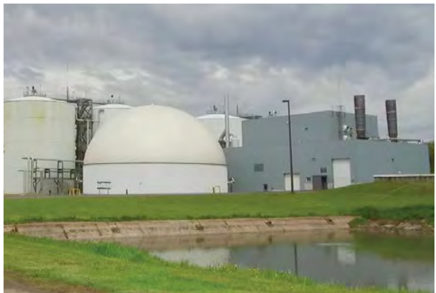
At Cavendish Farms on Prince Edward Island, digesters break down potato waste, producing biogas that fuels the boilers in the company's nearby French fry processing facility. (Image: Pat Martel/CBC)
